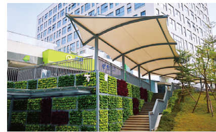
绿色出行，风雨连廊 Pedestrian and Cycling Paths, Covered Walkways
